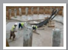
Foundations being laid for one of the 12 turbines the Lissett Wind Farm.
